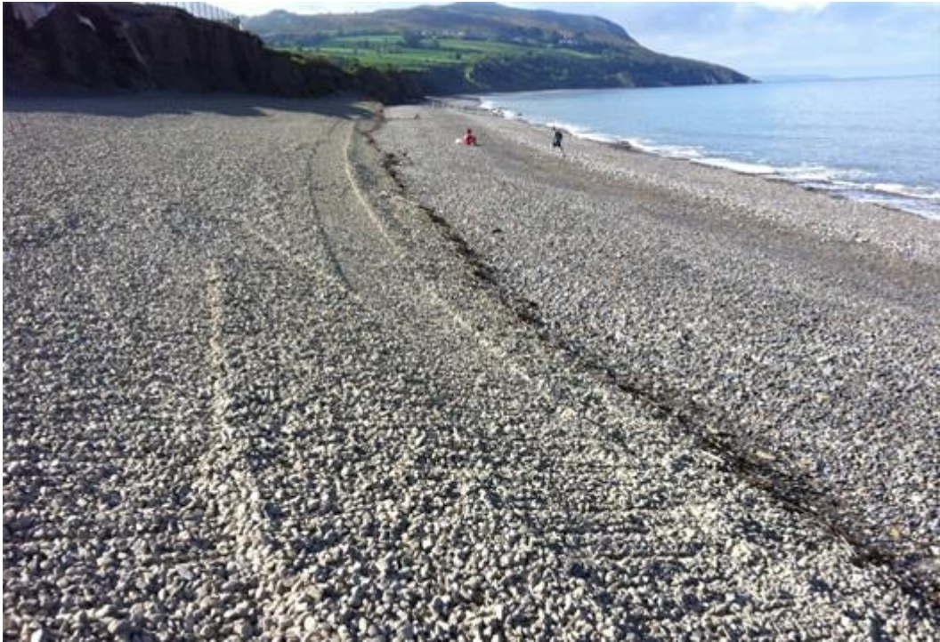
Figure 28: Completed beach nourishment works in the area between the revetment and the Gap Bridge. Site visit 25 May 2014
